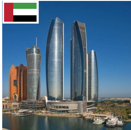
Etihad Towers Abu Dhabi UAE
