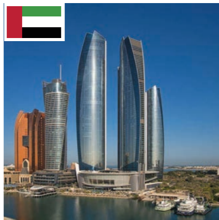
Etihad Towers Abu Dhabi UAE
