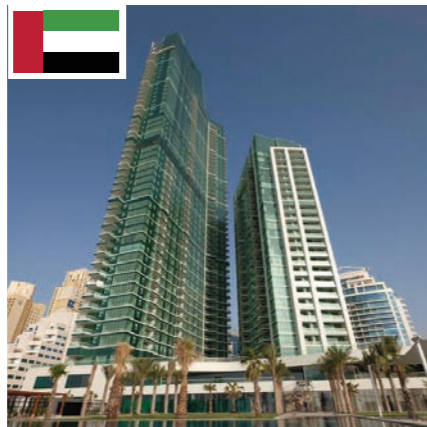
Al Bateen Tower Dubai UAE
